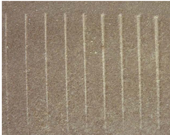
Figure 5: Oblique chisel grooves resulting from misalignment of chisel and stone surface
